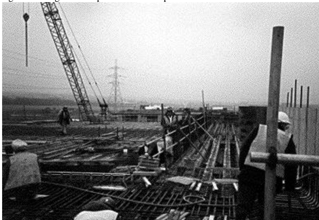
fig. A.1. Bridge surface prior to concrete pour.
